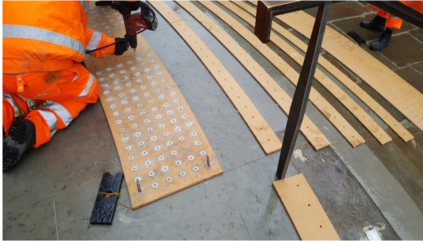
Setting Out & Pre-Drilling
