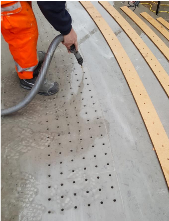
Cleaning Out Holes
